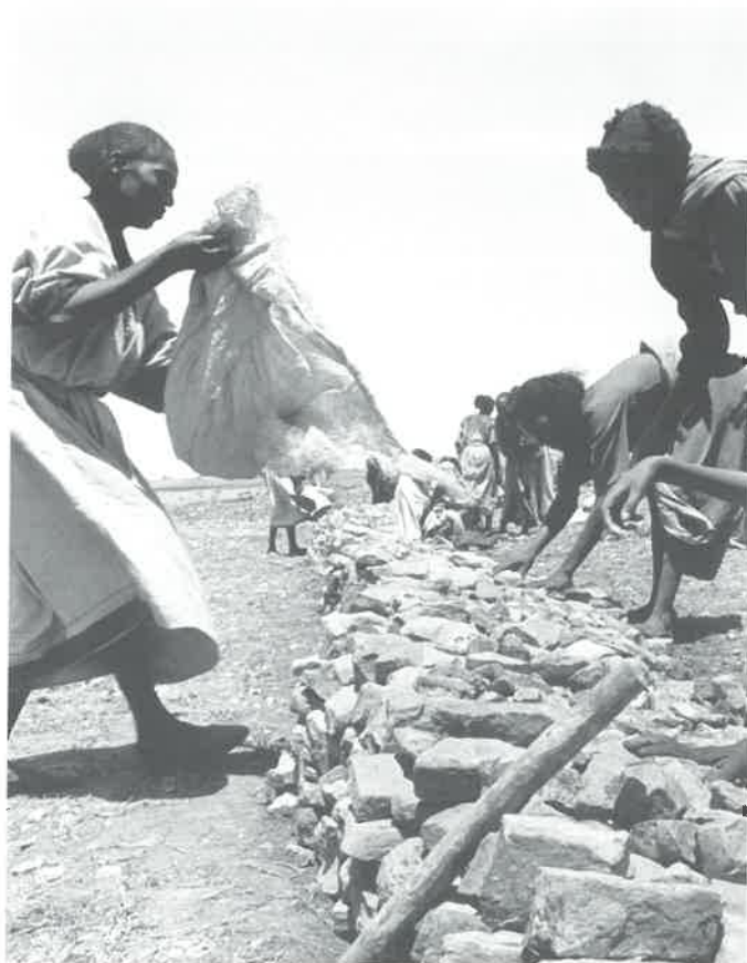
Terracing the land against soil erosion, Tigray, Ethiopia
